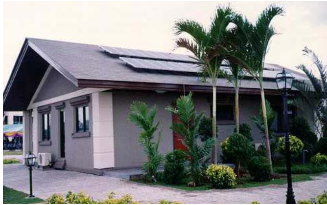
Figure 4: Vanadium Battery powered Solar Demonstration House in Thailand
